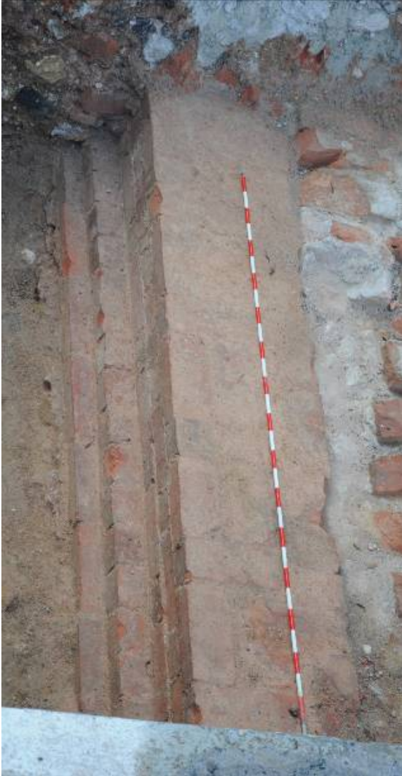
Structure underneath the Parade Ground probably associated with the rest room of the Central Police Station
